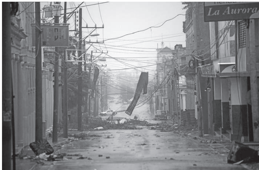
Debris covers a street as Hurricane Ian passes through Pinar del Rio, Cuba, Sept. 27. The entire island of Cuba is without power, following the destructive winds and flooding left in the wake of Hurricane Ian. Preliminary reports point to major damage in Pinar del Rio.
